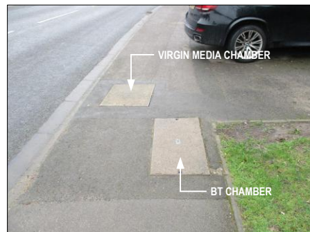
PHOTOGRAPH 2 EXISTING BT AND VIRGIN MEDIA CHAMBERS IN FOOTWAY ON GARDNER ROAD TO WEST OF ENTRANCE
